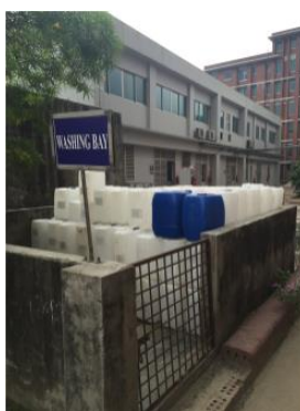
Picture 2: designated area to wash the empty chemical drums to remove the residues left inside these drums. The wastewater from the area to wash the empty drums is directly discharged into the receiving tank of the effluent treatment plant (see blue arrow).
